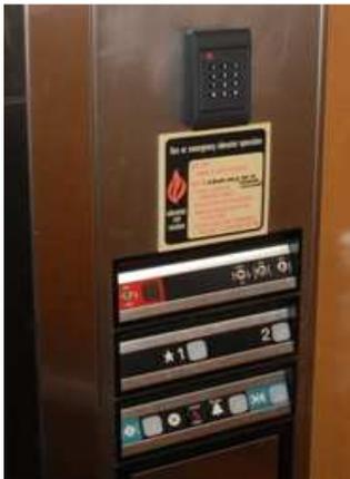
**Operating Modes** The DK-1025 can be used for Card + PIN, PIN + Card, Card Only or PIN Only. Mode selection is made by programming the host system, not by selection in the DK-1025.
